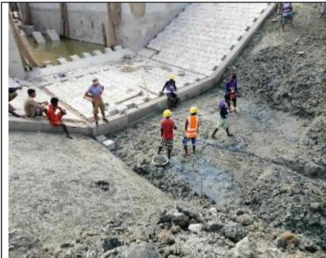
Figure 3-74: CC Blocks placing for loose apron (C/S) & slope of DS-01 in Polder 47/2
