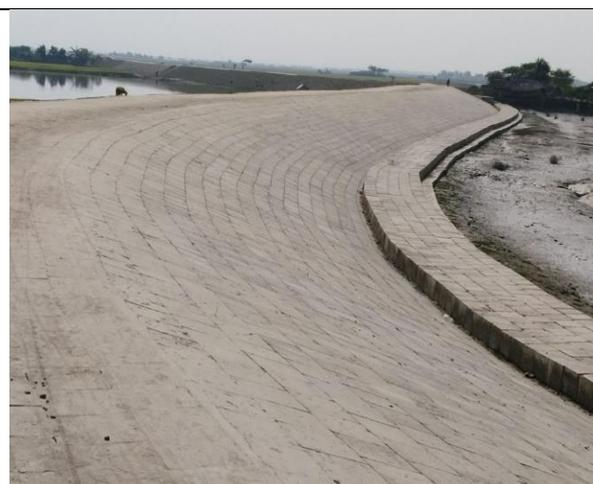
**Figure 3-42: Completed Slope Protection Works in Polder-32**
