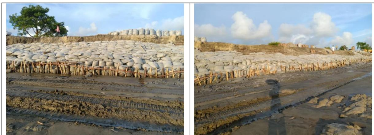
Figure 3-80: Emergency Work of Polder-48
