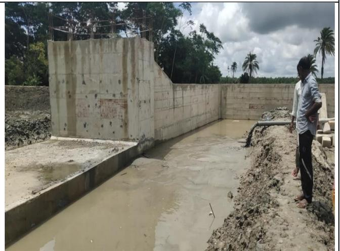
Figure 3-65: Backfilling with sand at DS-8 in Polder 41/1
